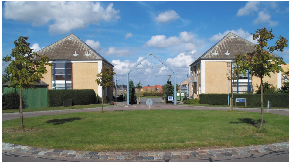
Figure 6.25 Development with iron entrance gate
